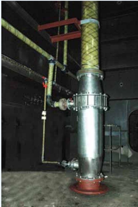
GLD™ unit installed in the ballast tank of a VLCC
